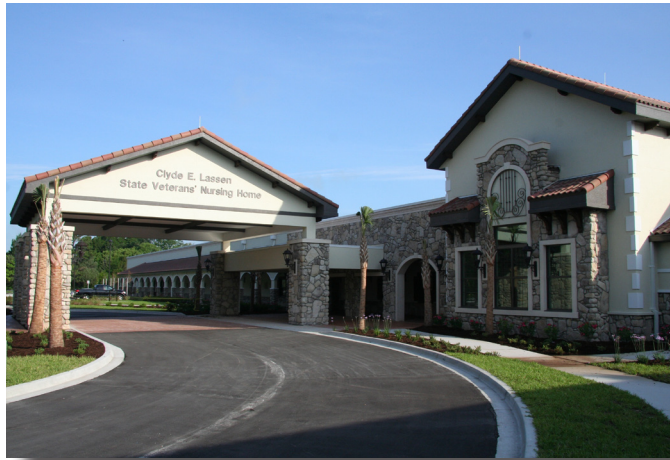
The Clyde E. Lassen State Veterans' Nursing Home in St. Augustine has been certified as LEED Gold by the U.S. Green Building Council. The 120-bed skilled nursing facility is the first Florida veterans' home to be named after a U.S. Navy veteran. Photo courtesy of Skanska.
